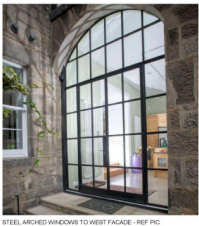
STEEL ARCHED WINDOWS TO WEST FACADE - REF PIC
